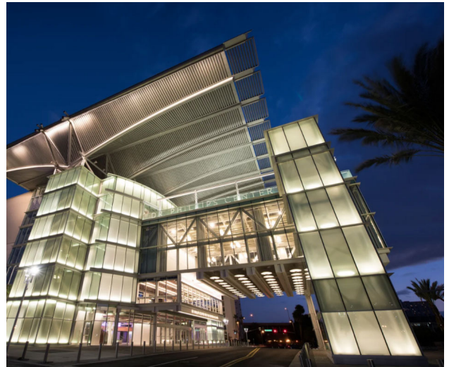
The Dr. Phillips Center for the Performing Arts concert hall is known as one of the city's most striking buildings
