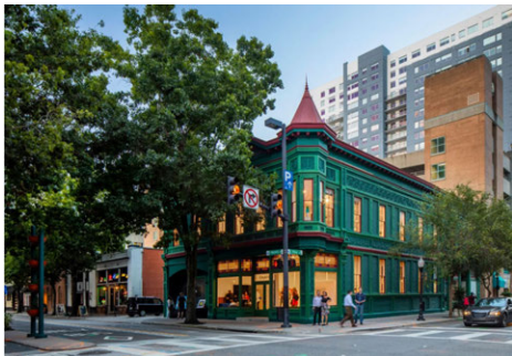
The Rogers Kiene Building in Downtown Orlando is one of the few remaining Victorian-era structures in the city, and is home to Orlando's eminent cultural venue CityArts Factory
