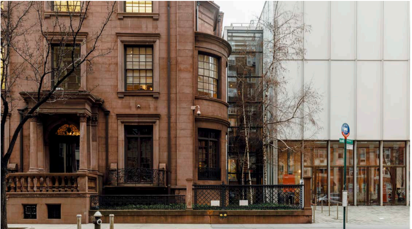
Above: The Morgan's extension (in white) stands in contrast to the original red-brick building
